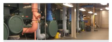
The plant provides a cooling capacity of 5,000 tons and a heating capacity of 49 MMBtu. Built with room for expansion, the CUP also houses the hospital's emergency generators and features:
