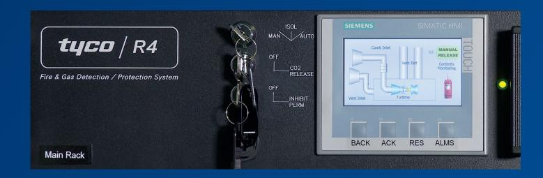
This HMI will provide individual graphical representations of the various fire zones along with individual status screens for each fire & gas field devices.
